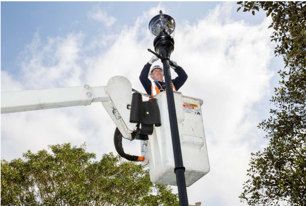
Left: installing LED lighting at Hollis Park.
